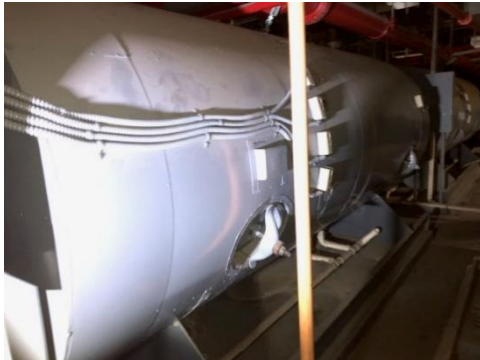
Figure 4-64 - Electric Boiler
