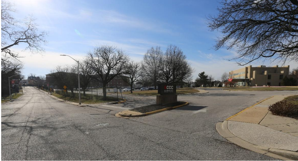
Figure 4-80 – View of the South Pavilion from the North Pavilion
