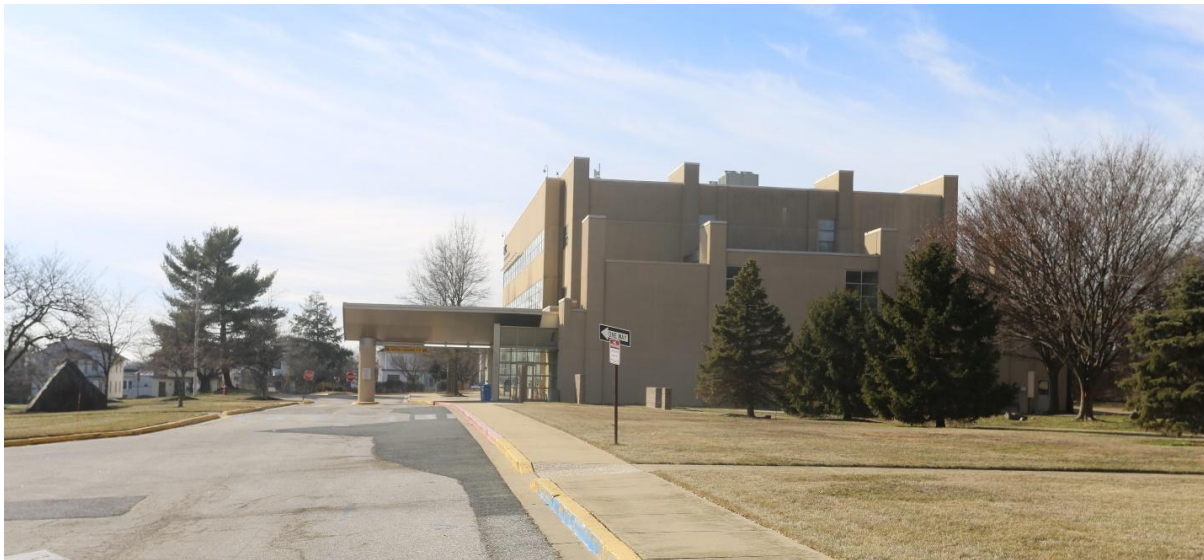
Figure 4-68 – South Pavilion exterior
