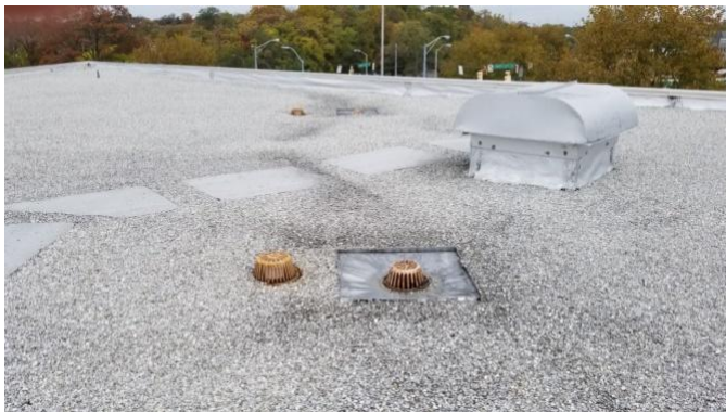
Figure 4-43 – Storm drainage system
