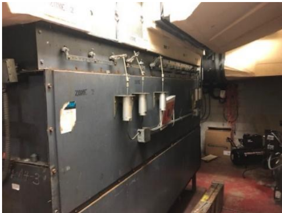
Figure 4-42 - Zone Dampers on Multizone Unit
