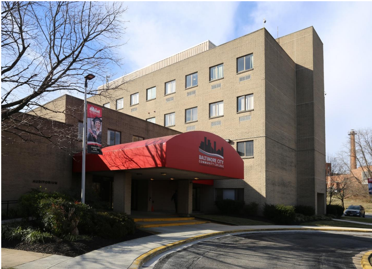
Figure 4-61 - West Pavilion entrance
