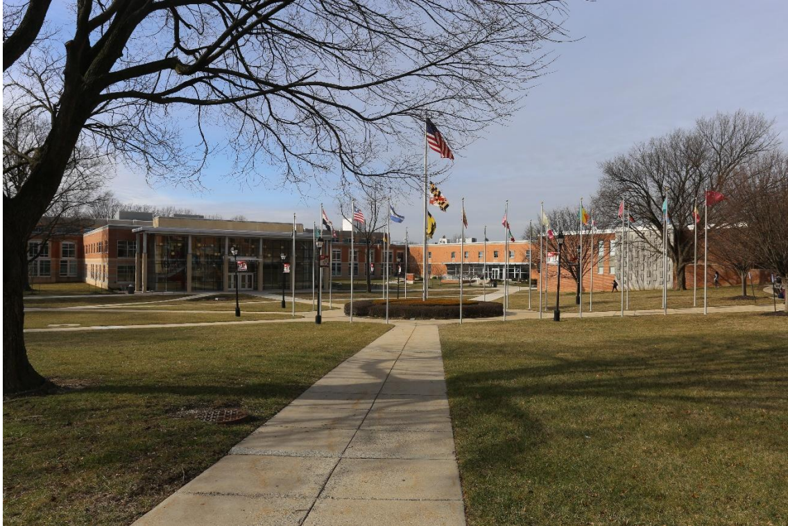
Figure 4-1 – Main Building from the center of campus
