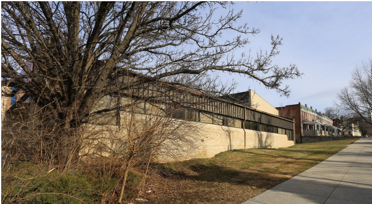
Figure 4-75 – North Pavilion exterior
