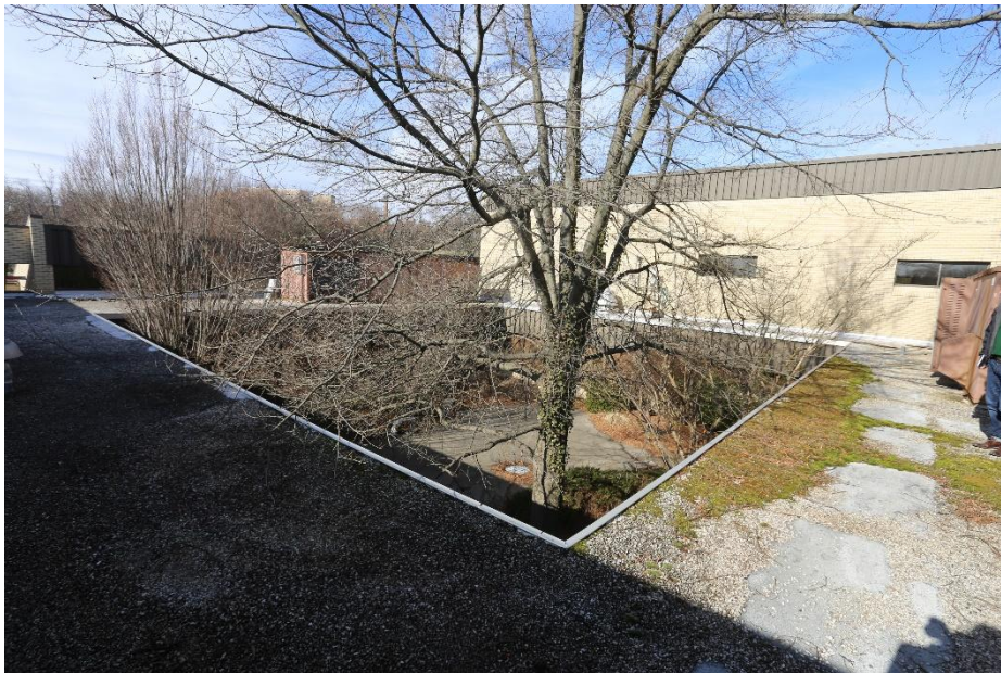
Figure 4-79 – Roof and courtyard
