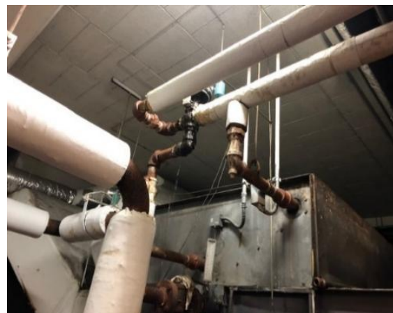
Figure 4-29 & Figure 4-30 – Library Piping Showing Missing Insulation and Leaks
