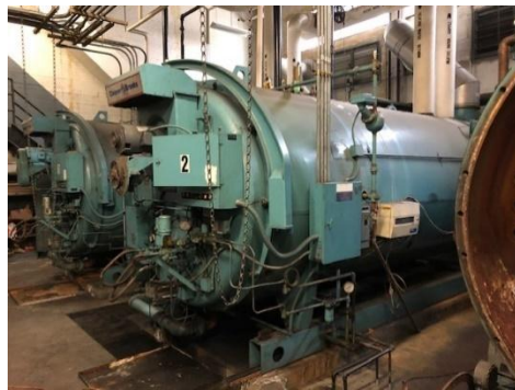
Figure 4-17 Fire Tube Boiler
